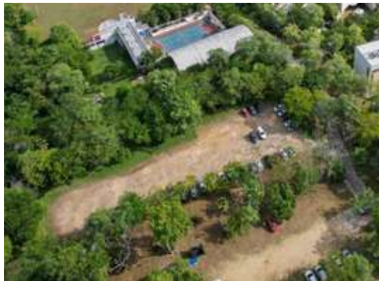
Parking lot A5 on natural terrain.
