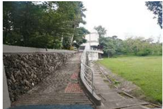
Access ramp to the Welfare Building.
