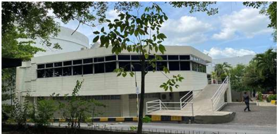
Illustration 9: Maloka Building – Technology Campus.
