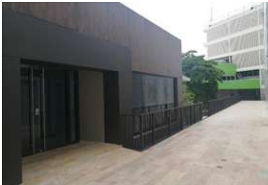
Bridge between Building A2 and Building Alcatraz.
